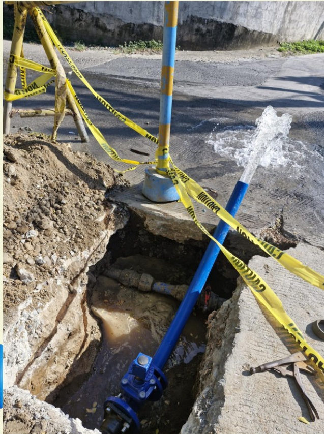
Energization of New Pipe Line at Brgy. San Jose Dike
