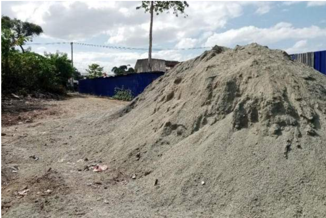
Figure 3-7 Stockyard for Delivered Aggregates
