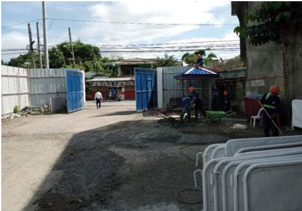
Figure 3-8 Workshop and Fabrication Yard
