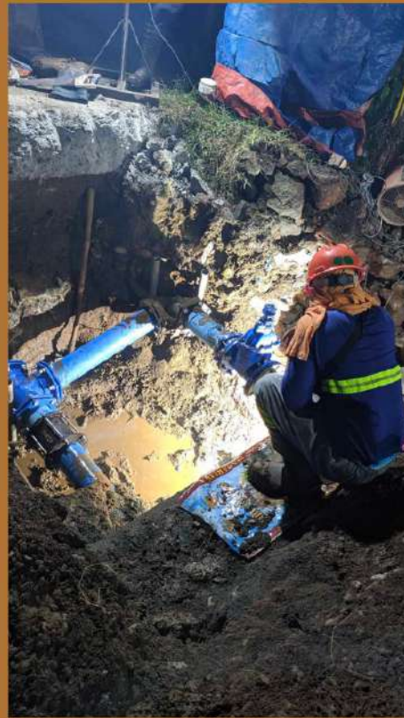
Part of interconnection activity 500 mm dia cement coated steel pipe at Brgy. Parulan
