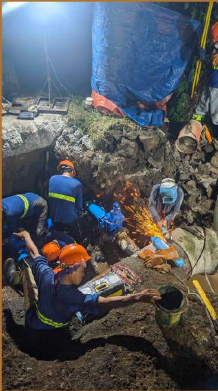
Part of interconnection activity 500 mm dia cement coated steel pipe at Brgy. Parulan
