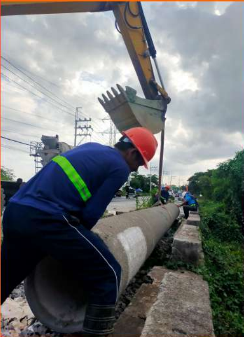
Installation of 500 mm dia Cement Coated Steel Pipe at Access Road Brgy. Parulan
