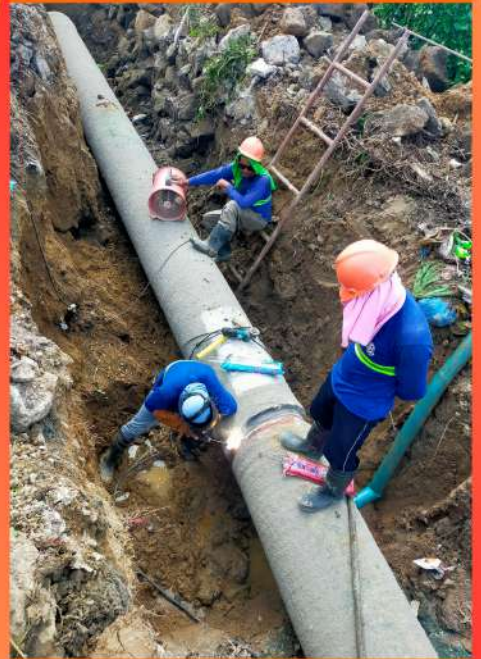
Installation of 500 mm dia Cement Coated Steel Pipe at Access Road Brgy. Parulan
