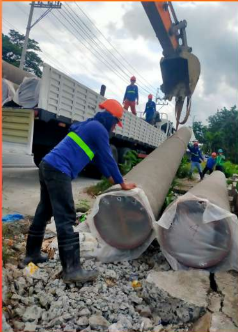
Installation of 500 mm dia Cement Coated Steel Pipe at Access Road Brgy. Parulan
