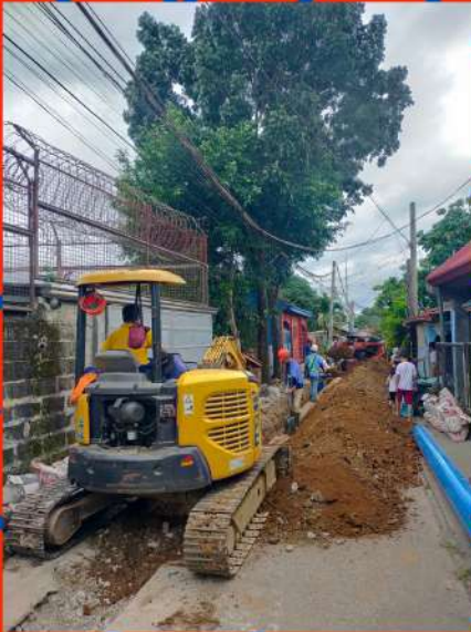
Brgy. Parulan Pipe Laying 250 mm dia
