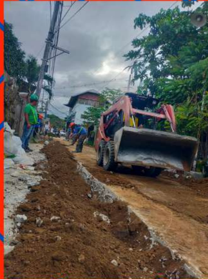
Brgy. Parulan Pipe Laying 250 mm dia
