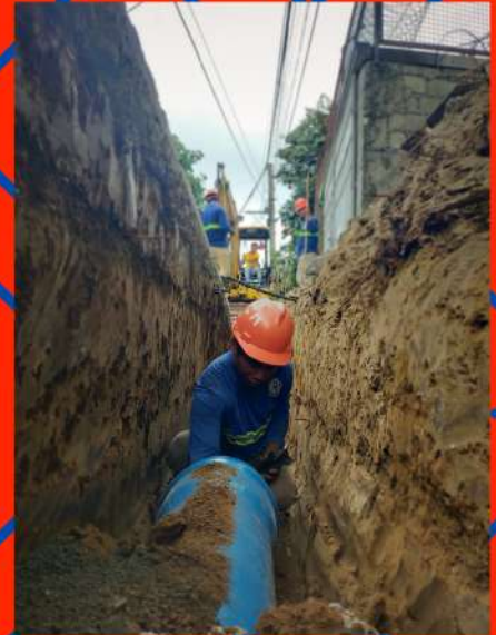
Brgy. Parulan Pipe Laying 250 mm dia
