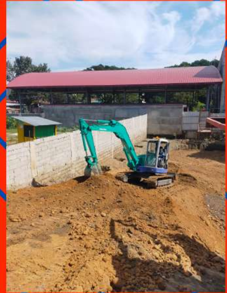
Backfilling Banga 1st Reservoir
