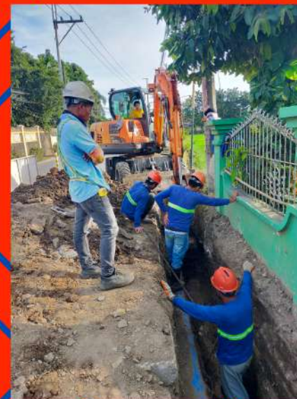
Brgy. San Jose Pipe Laying 300 mm dia
