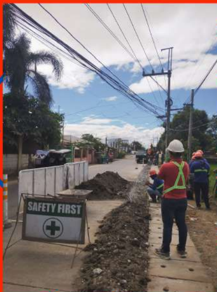
Brgy. San Jose Pipe Laying 300 mm dia
