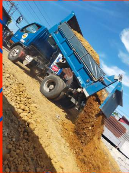
Backfilling Banga 1st Reservoir
