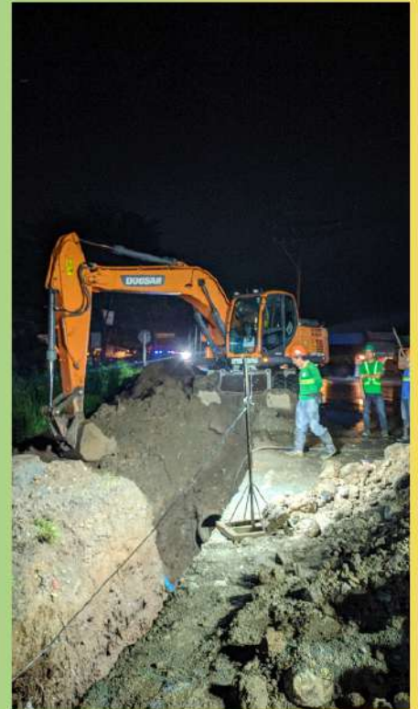
Interconnection of 500 mm dia. Cement Coated Steel Pipe at Brgy. Parulan prior to energization of additional water supply for Brgy. Banga 1st, Banga 2nd and Bagong Silang.
