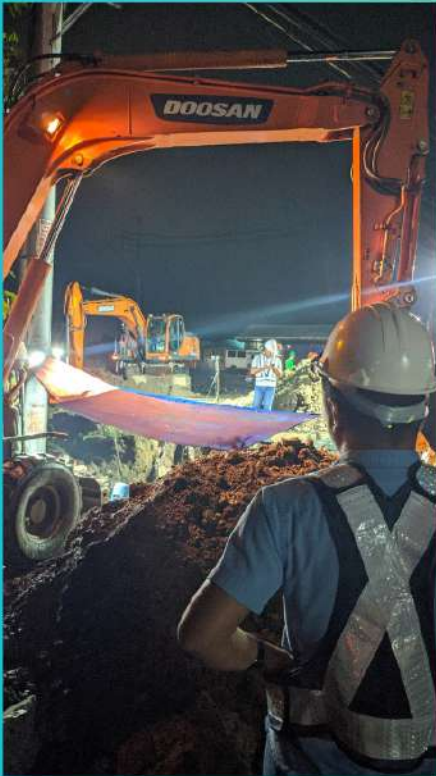
Interconnection of 500 mm dia. Cement Coated Steel Pipe at Brgy. Parulan prior to energization of additional water supply for Brgy. Banga 1st, Banga 2nd and Bagong Silang.
