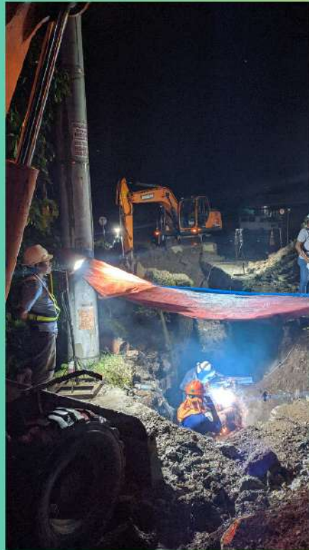
Interconnection of 500 mm dia. Cement Coated Steel Pipe at Brgy. Parulan prior to energization of additional water supply for Brgy. Banga 1st, Banga 2nd and Bagong Silang.
