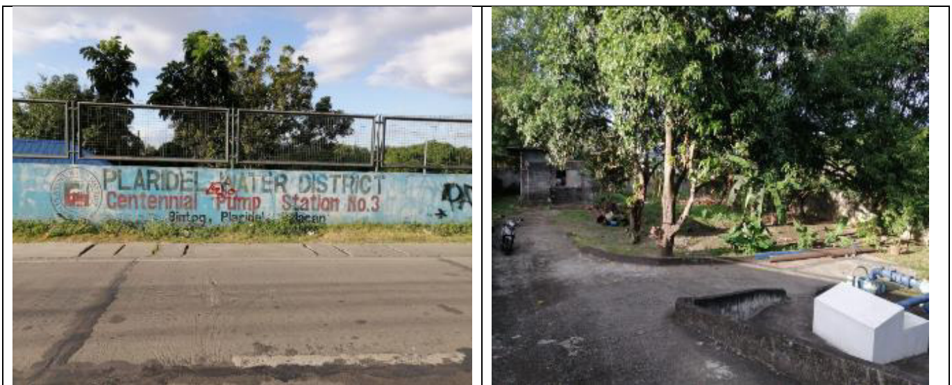
Proposed Office Building/Motorpool/Warehouse will be located in the existing compound of Centennial Pump Station No. 3 in Bintog, Plaridel, Bulacan
